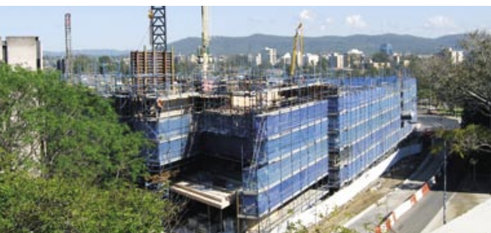
6th Floor form work being added to the new GPN4 Building
